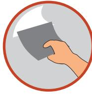
Smoothen the surface by applying thin coats of putty to fill in all the dents. Allow the putty to dry overnight.
